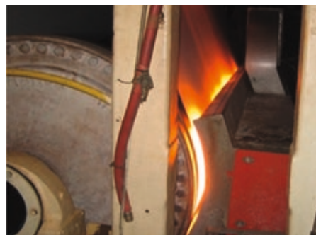
Fig. 16: Space-saving installation of an eNIR emitter with curved infrared lamps adapted to drying cylinders for optimum energy input into the web. Moist areas can be recognized, where the lamps shine with higher power
